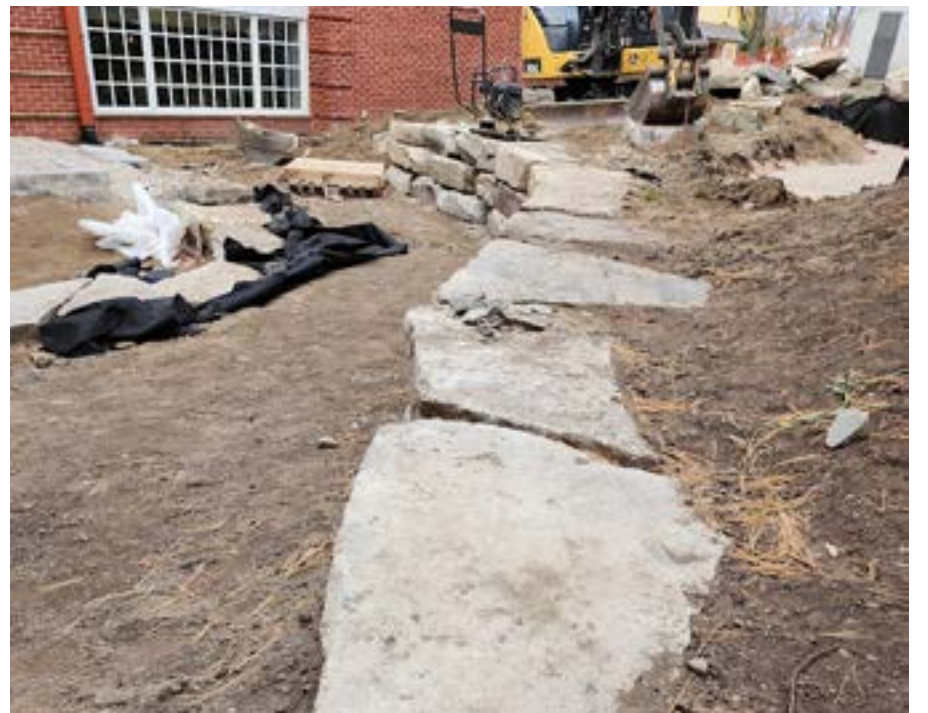
Construction of the amphitheater opening Summer 2024
